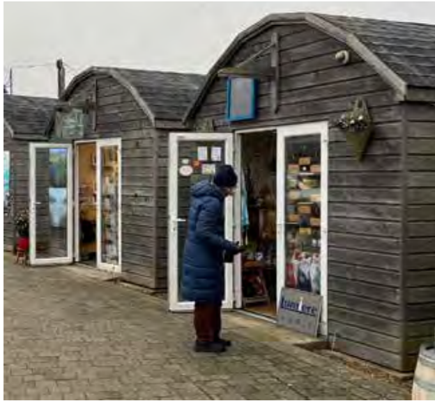
Sunken down + gravel drainage
