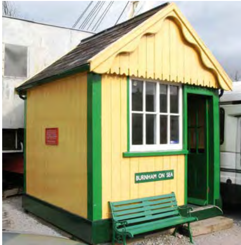
Burnham on sea signal box Size: 3x3m
